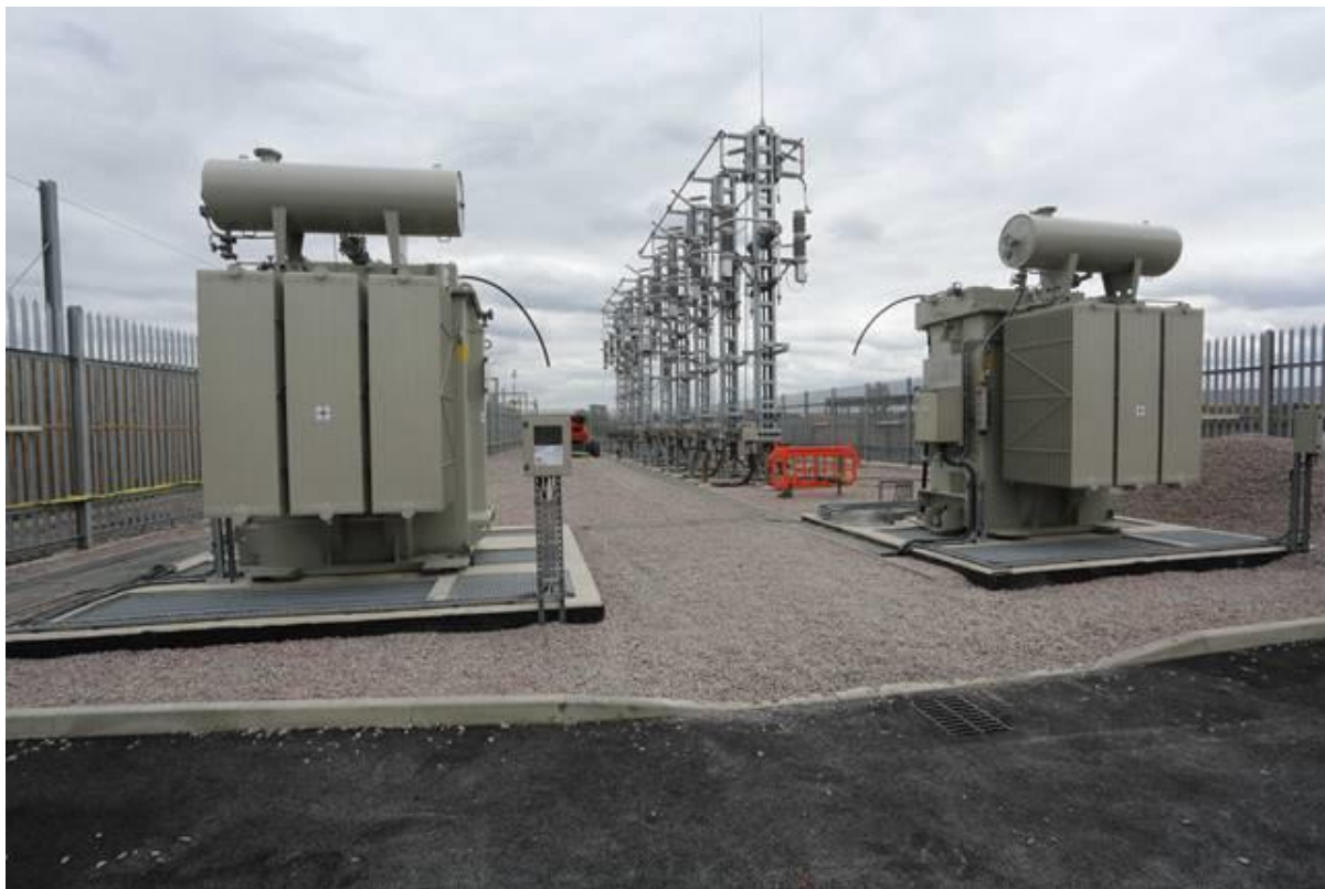
FIGURE 4 AUTOTRANSFORMER STATION
